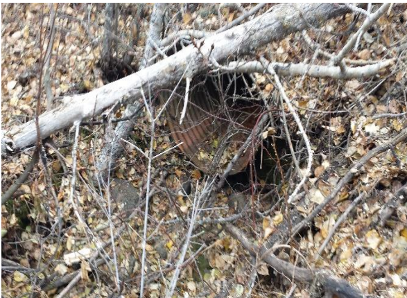
Photo 13: Crossing 2 culvert outlet.
