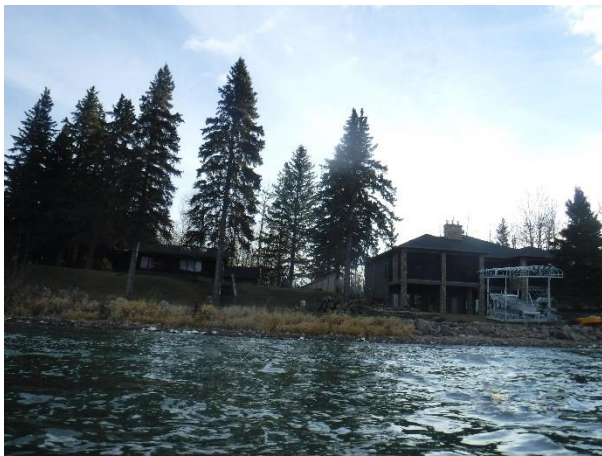
Photo 3: Shoreline disturbance including buildings, lawns, rock placement and vegetation clearing within Reach 2.
