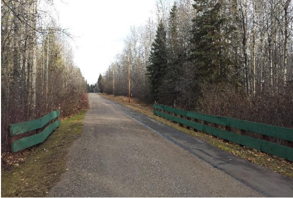
Photo 11: Crossing 2 road view.
