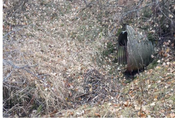
Photo 12: Crossing 2 culvert inlet.
