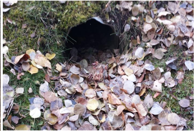
Photo 8: Crossing 1 culvert inlet.
